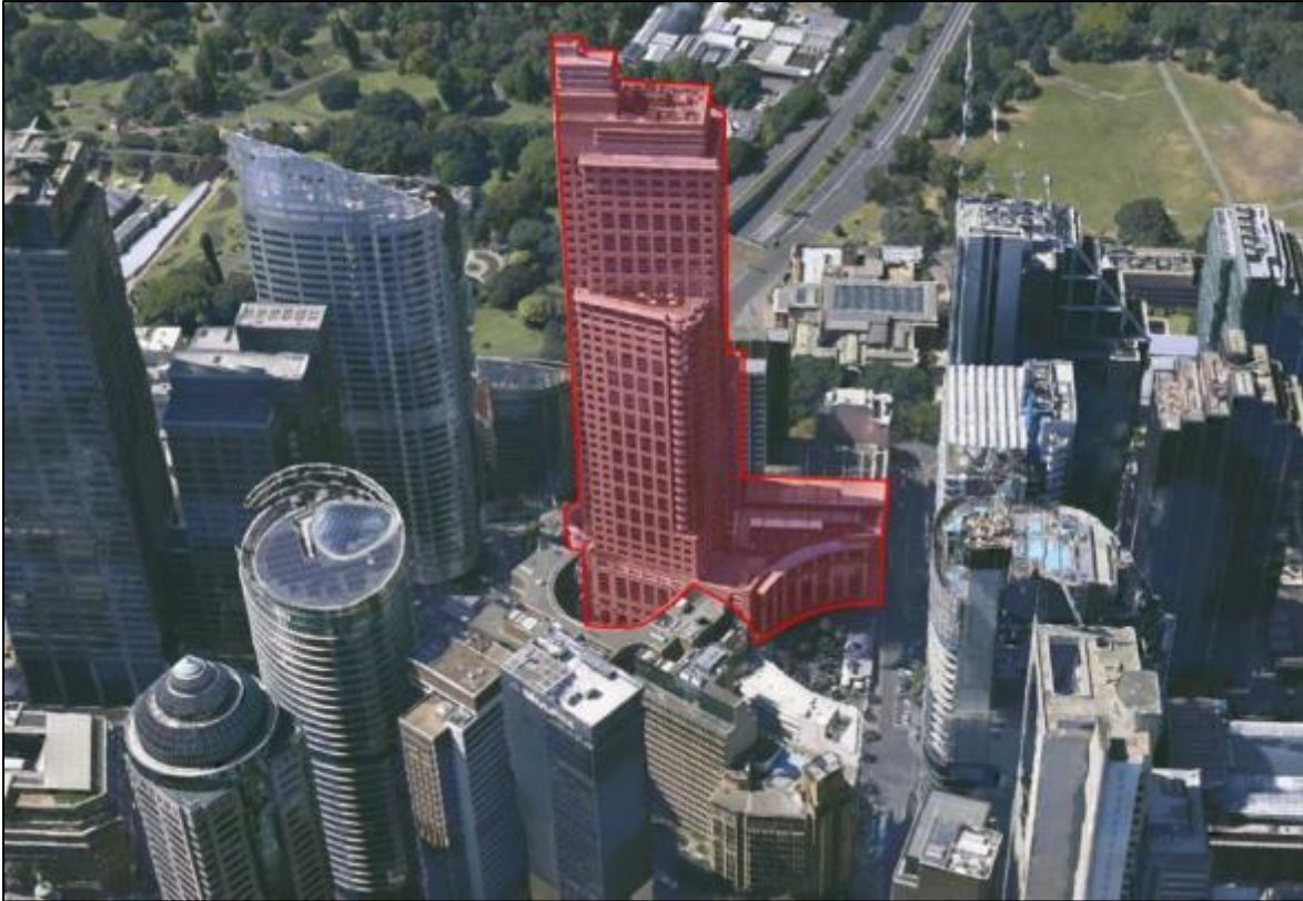
Figure 2: Oblique aerial of the subject site, looking east
