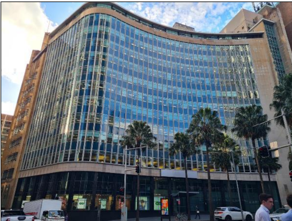
Figure 12: Qantas House to the south-west of the site, looking west from Hunter Street
