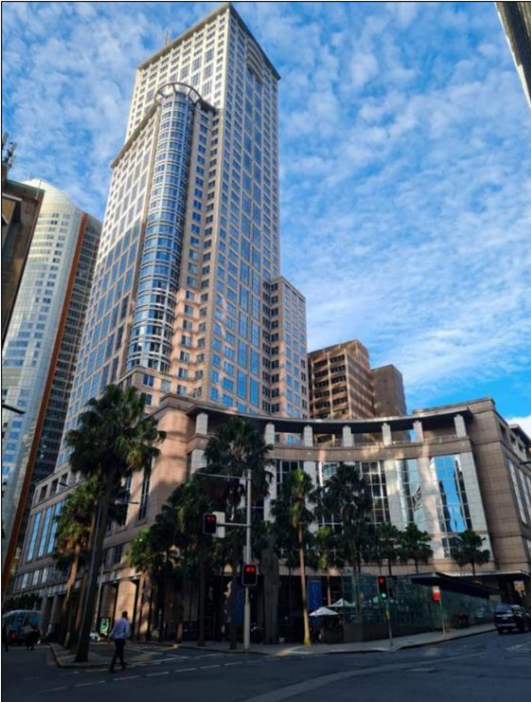
Figure 5: Chifley Square, Chifley South podium and Chifley North viewed from the corner of Hunter and Phillip Streets, looking north-east
