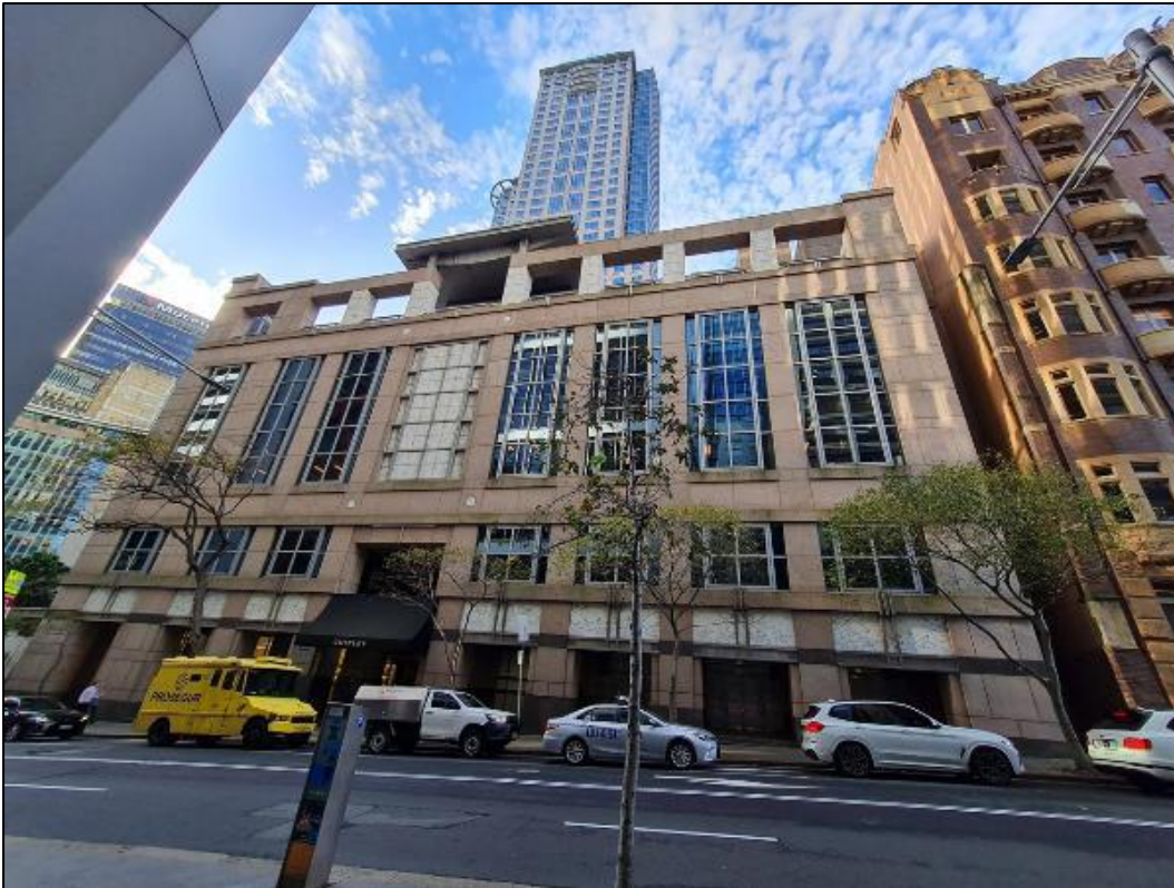
Figure 6: Chifley South podium viewed from Hunter Street, looking north
