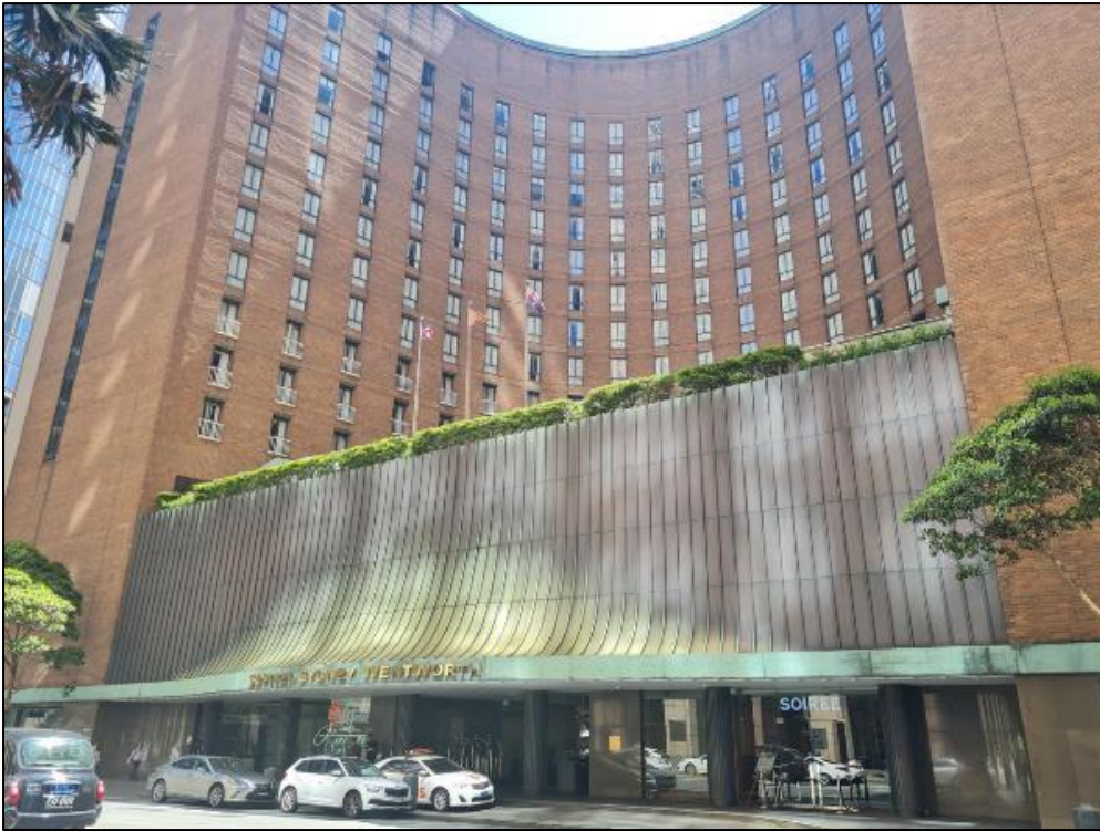
Figure 11: Sofitel Wentworth Hotel directly to the west of the site, looking west from Phillip Street
